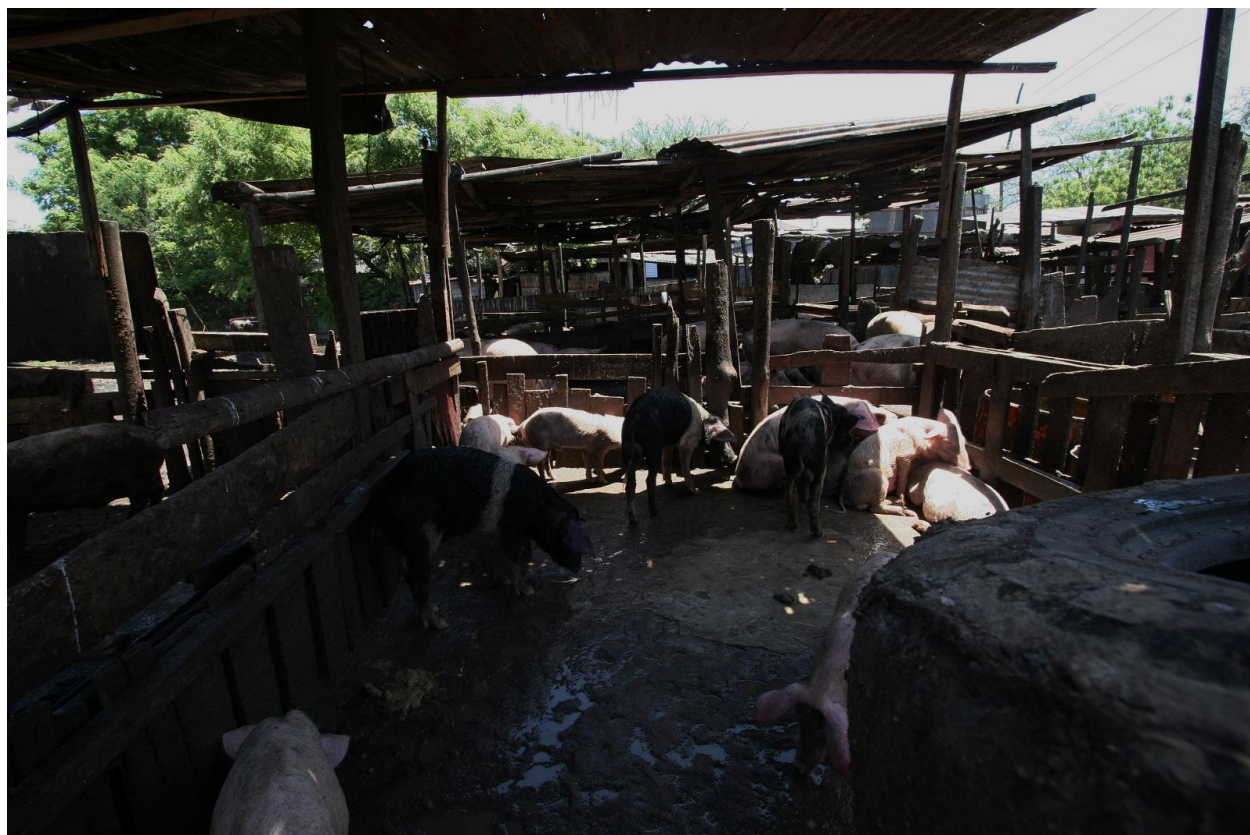
Figure 1. Unhygienic and poorly constructed pig housing in a Dar es Salaam suburb
